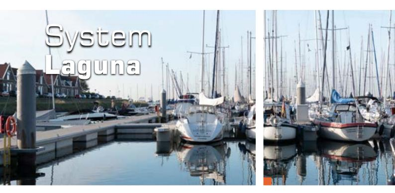
System Laguna is a modern sustainable floating modular pontoon system with a virtually maintenance-free seawater-resistant aluminum frame that is suitable for use in protected harbor locations and areas with harsh climatic conditions.
